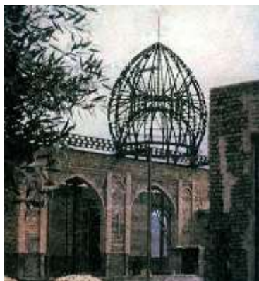
Figure 11: The dome of a mosque in Qom, Kashan way, although the dome next to the skin, but the idea implemented with new materials and traditional design.
