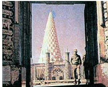
Figure 12: Burj al Seljuk period in Hamedan, the Dome of the rack and a dozen cracks or dodecahedron.
