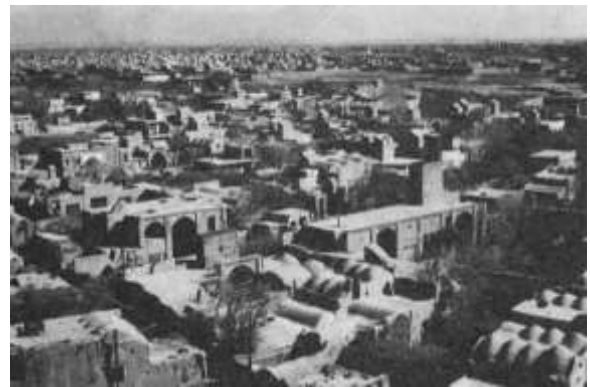
Figure 2: The central courtyard of the building, the ceiling of the dome and the wind short one-way Meibod A prominent feature of the city landscape on the edge of Kavir Yazd province
