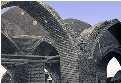
Figure 10: How Kolonbeh the arch at the mosque of Imam Ali (AS) in Yazd.
